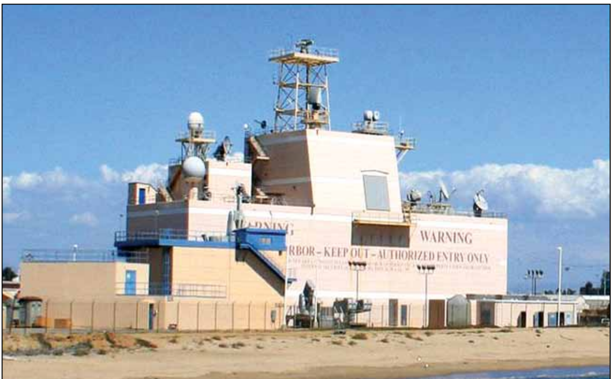
Figure 8. SWEF with the VSR Installed
