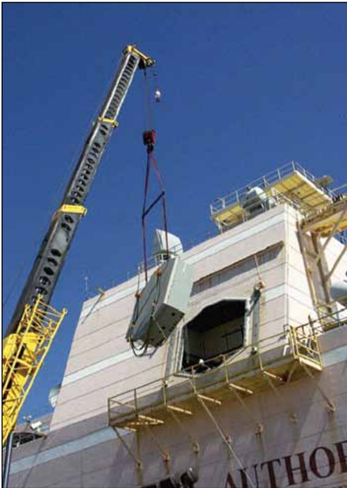
Figure 5. SPY-1A Array Being Uninstalled from the SWEF
