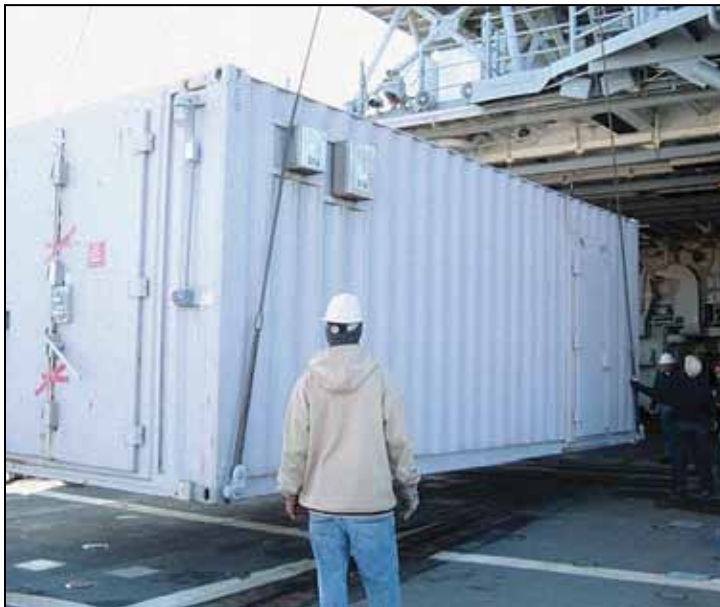
Figure 4. MFR Signal-Processing Enclosure Being Installed on SDTS
