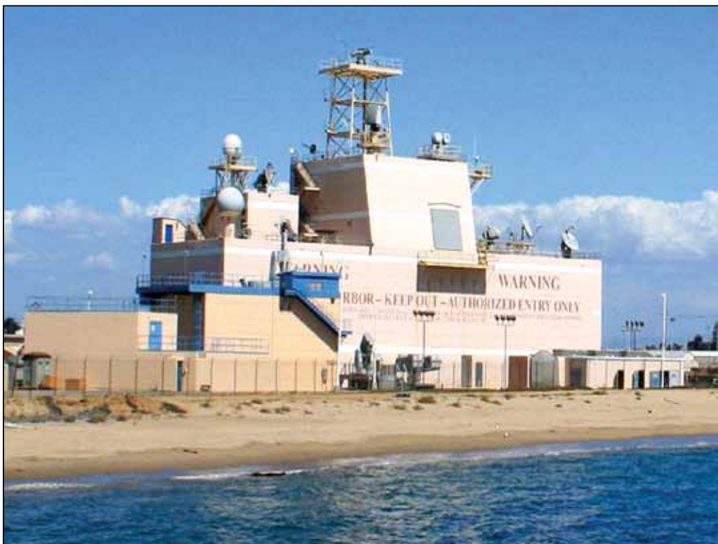
Figure 5. VSR Surface Warfare Engineering Facility Installation
