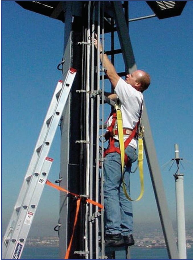
Figure 1. X-Band RAM Installation on USS Ronald Reagan (CVN 76) Stubmast
