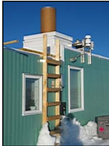
Exterior of "Green House" with roof penetration for SUV-150B optics
