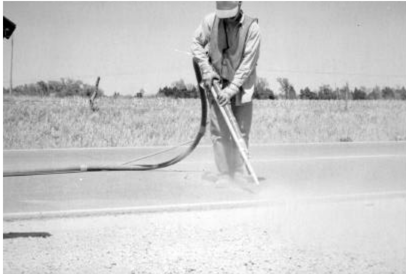
Figure 19. Sandblasting wand with wooden guide attached.
