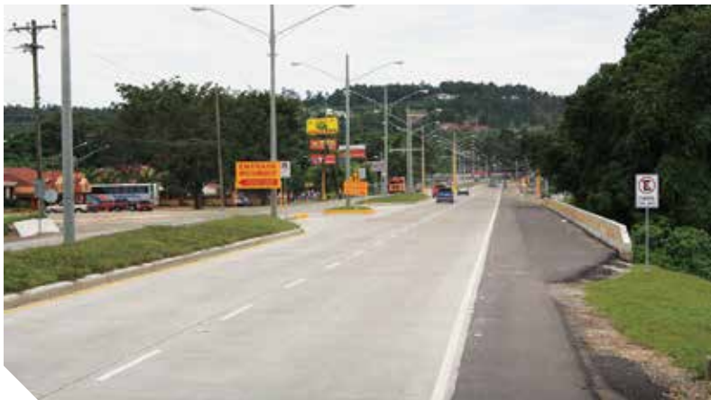
A section of the improved CA-5 highway is ready.
