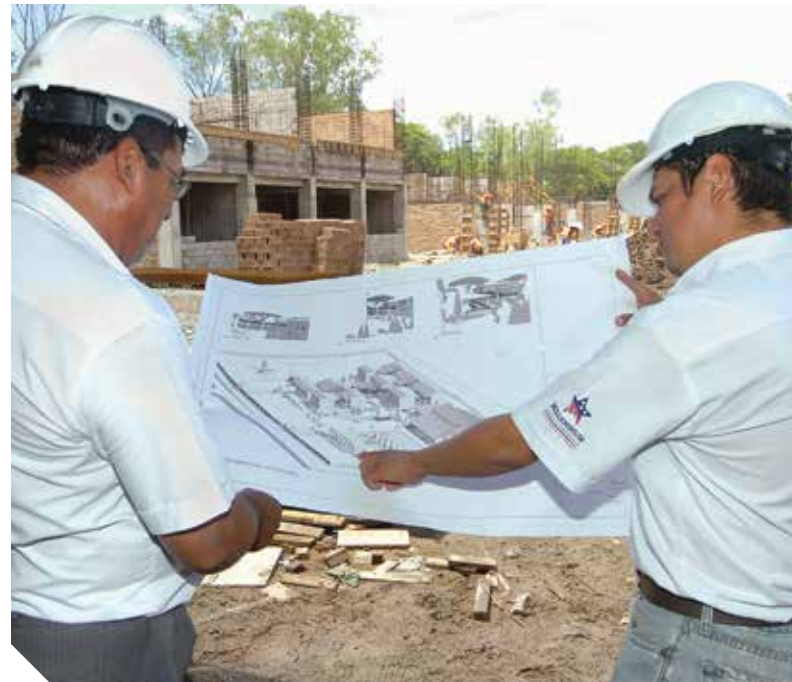
MCC funded the construction of the Technological Institute in Chalatenango, a state-of-the-art technical and vocational facility.
