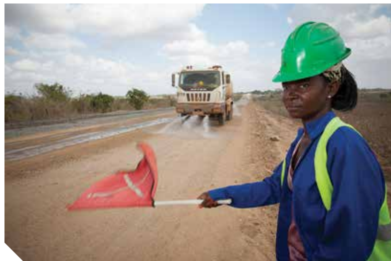
Road construction, Mozambique
