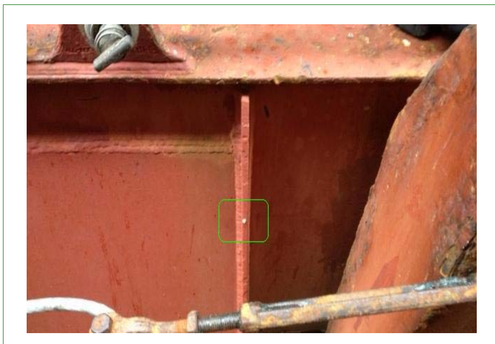
FIGURE 3-3-4: AGM Eggs Found Between Two Bays on a Support Beam Near a Cargo Hold Opening
