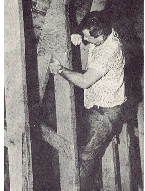
FIGURE D-11 Examining Grain Storage Bulkhead Supports
