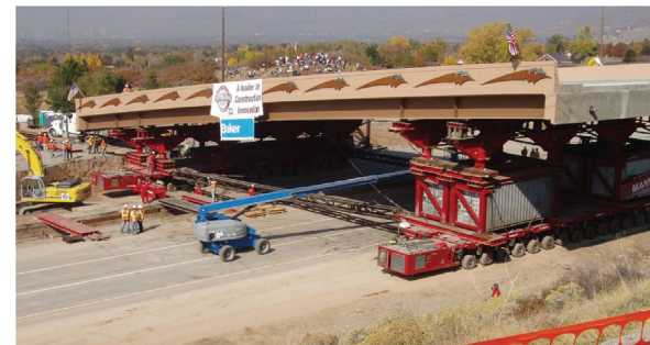
Moving the superstructure using SPMTs.
