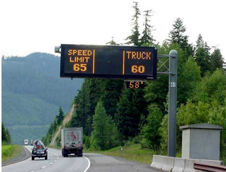
Figure 3. Variable Speed Limit Sign over Steven's Pass on US -2 in Washington State (Source: Washington DOT)
