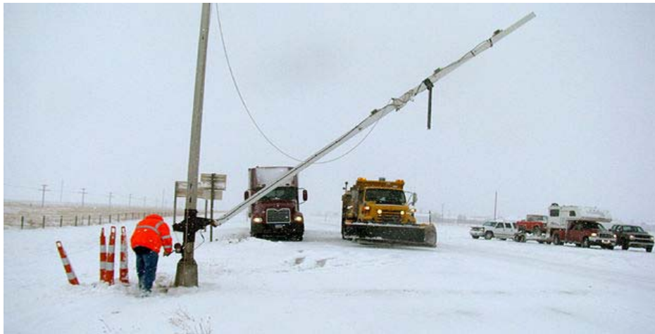
Figure 4. Example of a Gate Arm Used to Control Access to Sections of Highways in Wyoming (Source: Wyoming DOT)
