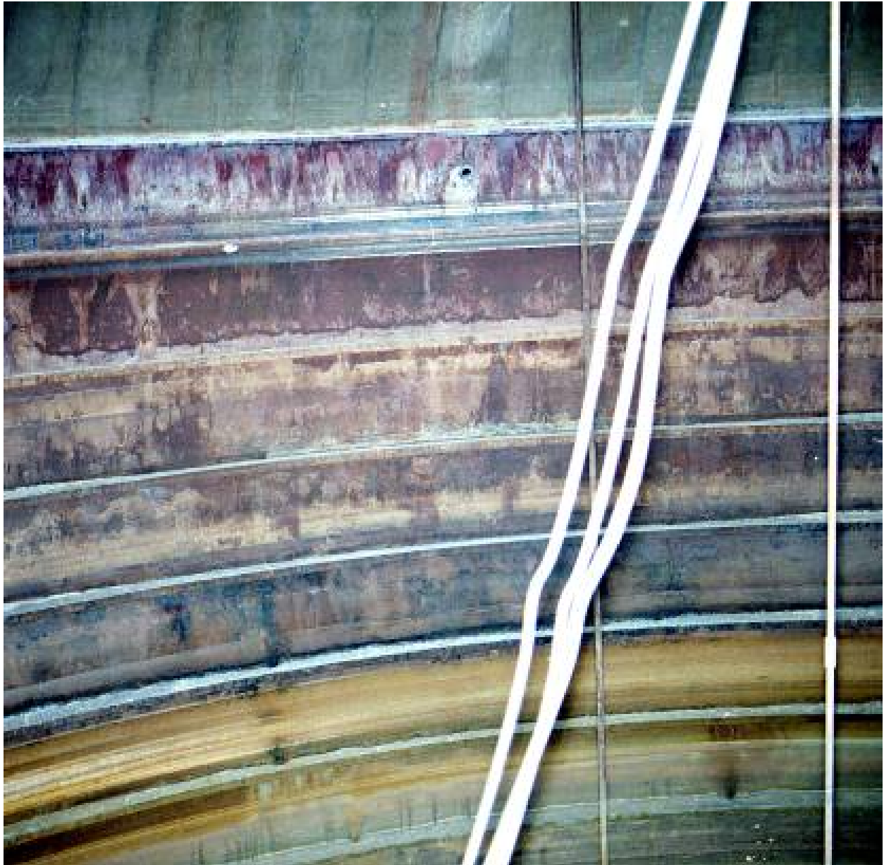
Figure 5.5-6. Tank 241-SX-110 Interior Wall (February 20, 1987)
