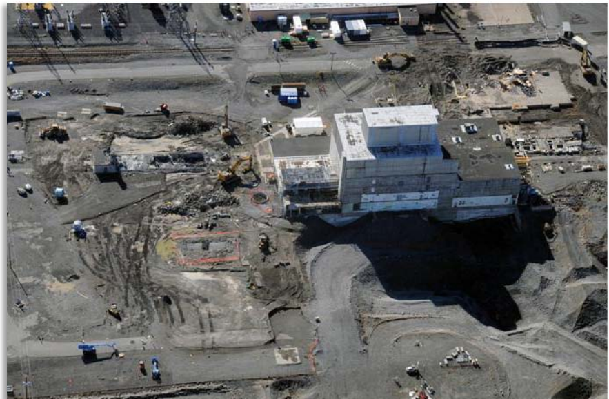
105KE Demolition & Remediation Sites
