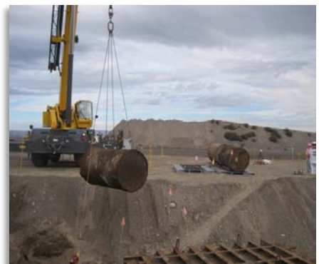
Culvert Removal
