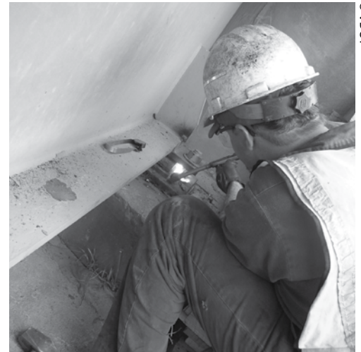
Work is done on a bearing device to facilitate the proper expansion and contraction of a bridge.
