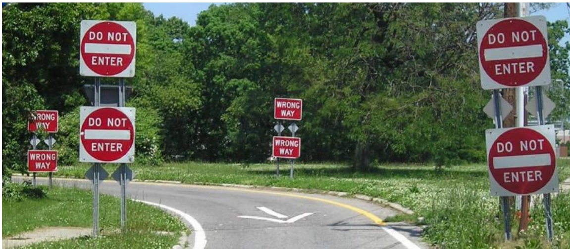
Figure 17. Double-posted “Do Not Enter” and “Wrong Way” signs on an exit ramp. (Courtesy of the New York State Department of Transportation).
