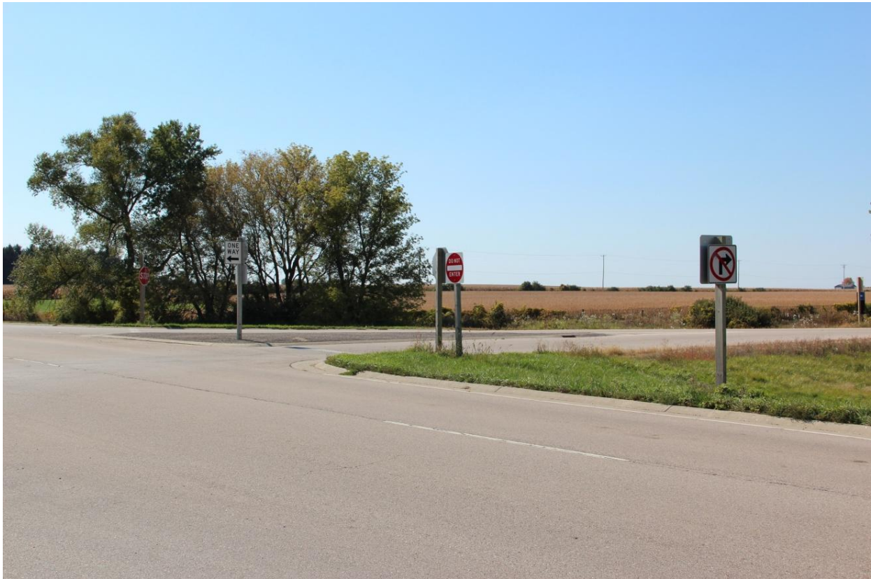
Figure 10. Possible wrong-way driver entry location for the Beloit, Wisconsin, collision.
