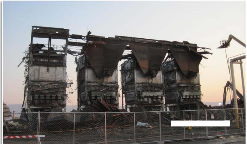
284W Power House Demolition
