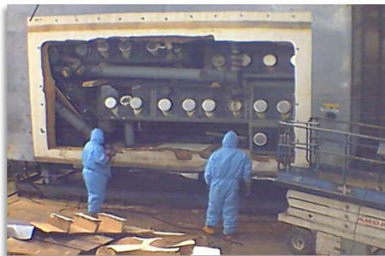
Large TRUM Waste FRP Being Cut Open at PFNW
