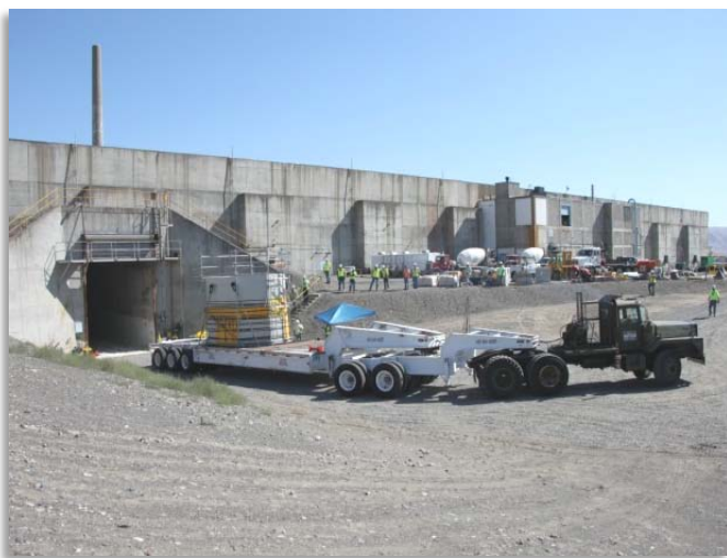
Tank D-10 is removed from U Canyon
