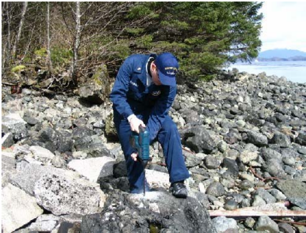
Ensign Matthew Glazewski of NOAA Ship FAIRWEATHER drills to establish a benchmark on Noyes Island, AK.
