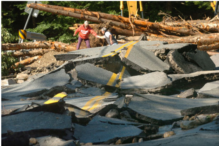
Box Figure 3.2. Hurricane Irene damage on Route 4 near Killington, Vermont. Source: Vyto Starinkas, Rutland (Vt.) Herald, via AP.
