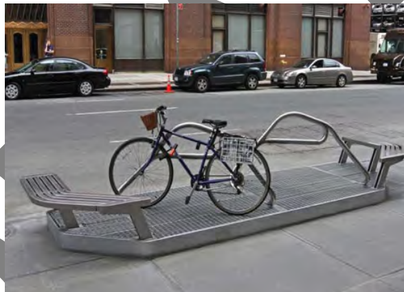
Figure 4.10. Raised Ventilation Grates in New York City. Source: MTA New York City Transit.
