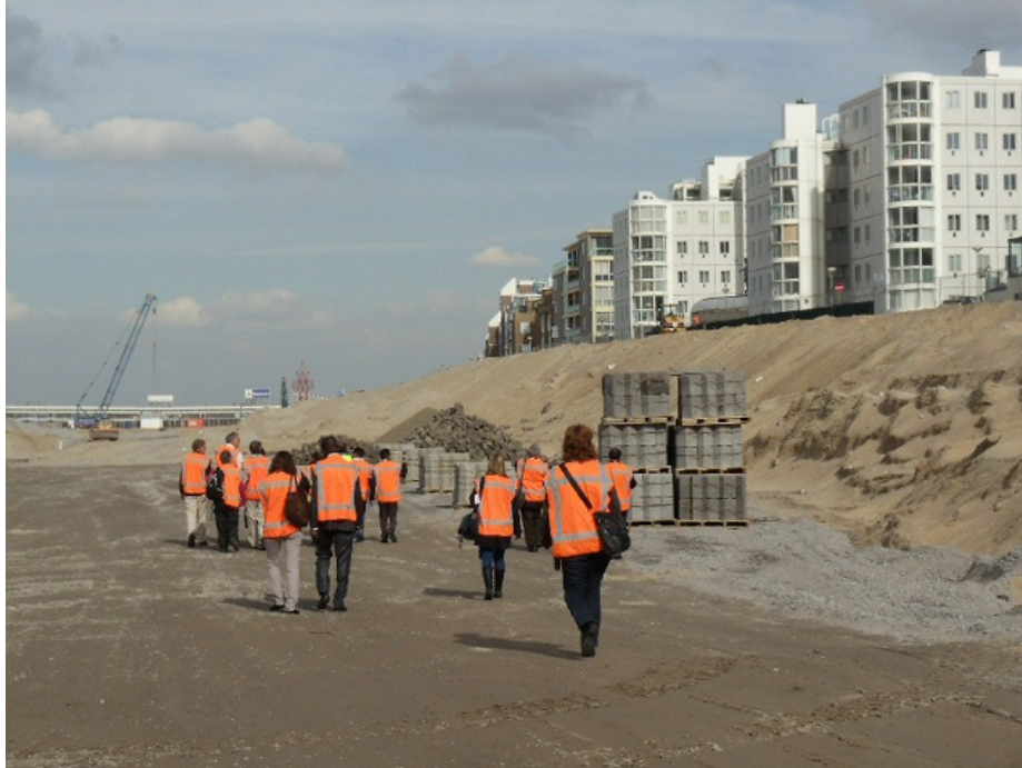
Figure 4.6. Raising and strengthening the levees in Scheveningen, the Netherlands. Notice the buildings on top of the structure. (Photo: V. Gornitz)
