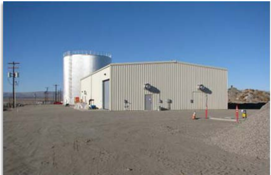
New 100K Area Water Plant
