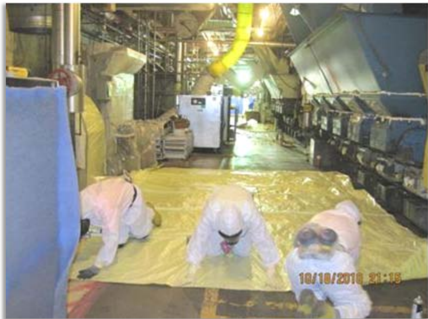
284E Powerhouse Asbestos Removal Preparations
