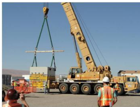
Offloading the D-10 Tank package at the Central Waste Complex
