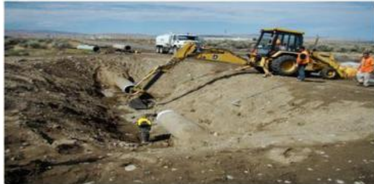
24-inch water line work at 200W
