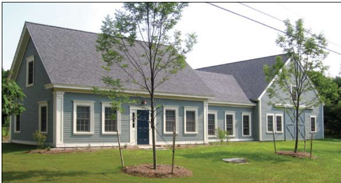
Figure VII.5. The Alheim Commons provides housing for visiting researchers, educators and resource managers.
