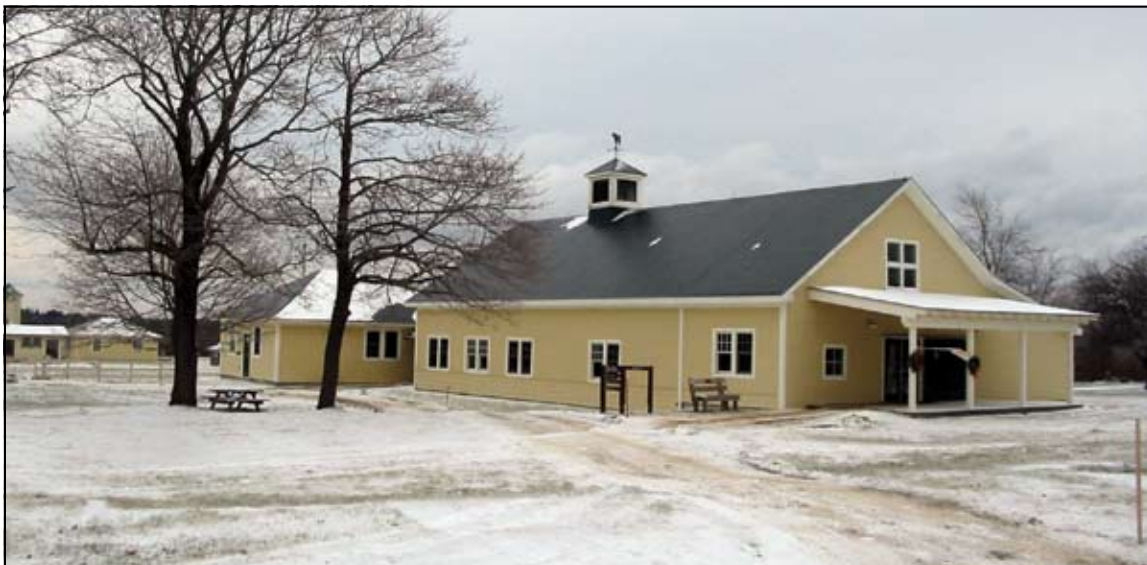
Figure V.1 The Maine Coastal Ecology Center, a 6,000-square-foot research and education facility, opened in 2001.
