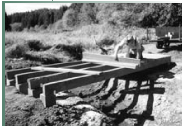
Maintenance staff constructs trail bridge
