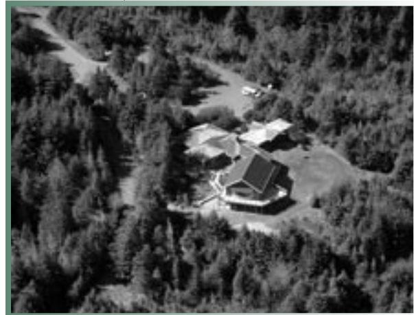
South Slough NERR Interpretive Center
