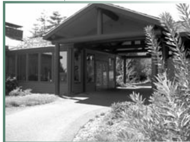
South Slough NERR Interpretive Center
