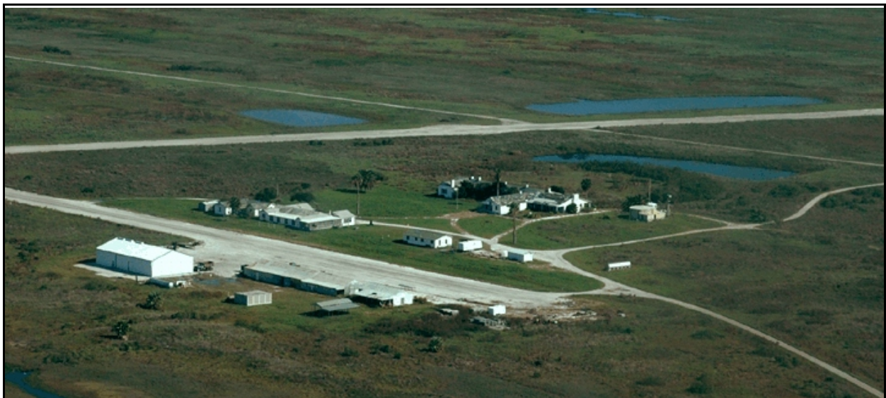
Figure 25. Wynne Ranch complex on Matagorda Island.
