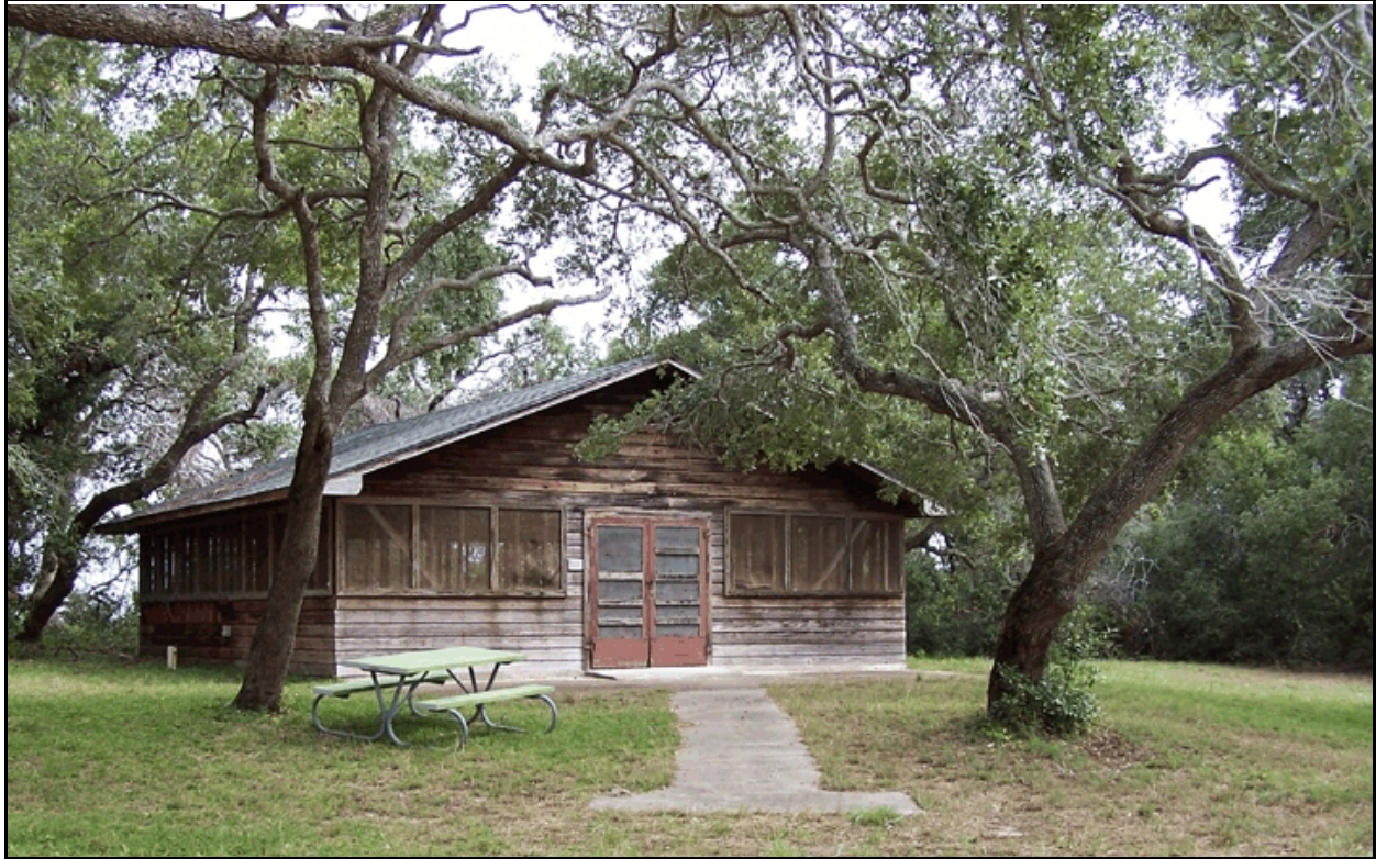
Figure 24. Covered picnic shelter at the ANWR Youth Environmental Training Center.
