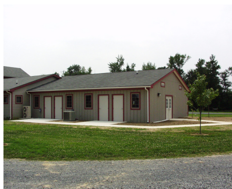
Figure VI-3. Phase I Addition.
