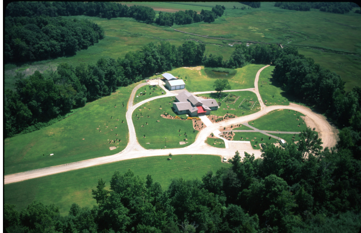
Figure II-5. Aerial photo of the Lower St. Jones River Reserve Component.
