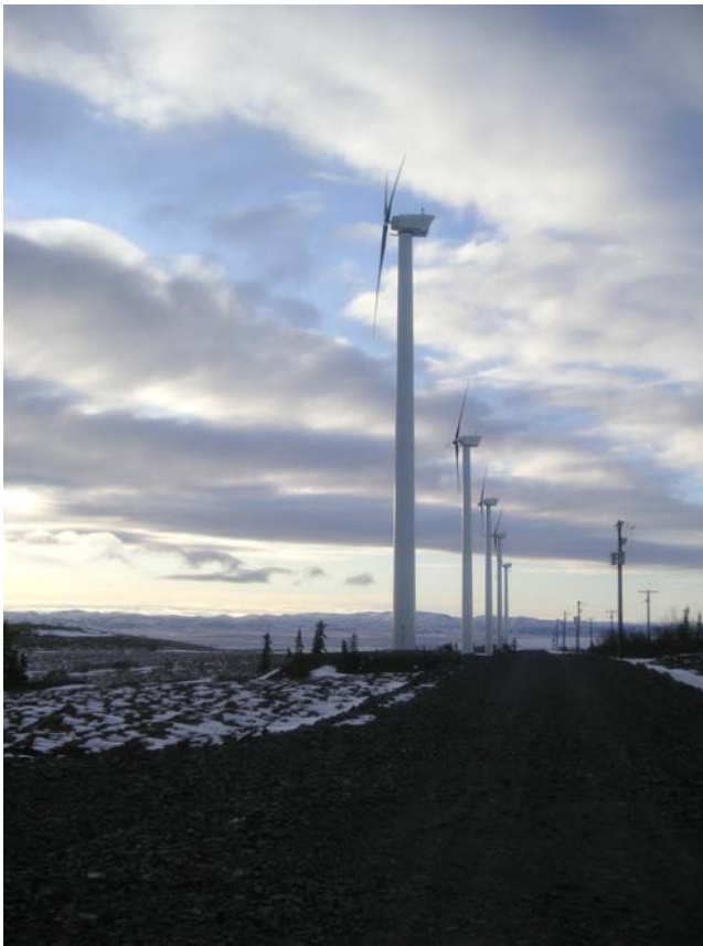
Wind Turbines supplying 30 Percent of Unalakleet's energy needs, partially funded by the Norton Sound Economic Development Corp. (CDQ group)
