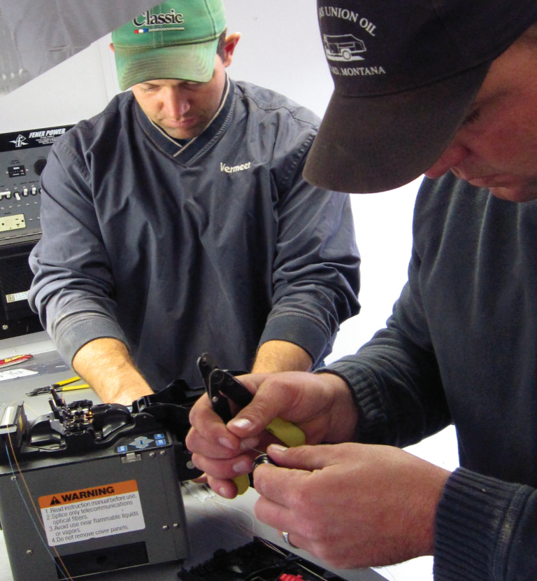
Triangle Communications field technicians splice fiber-optic cable.
