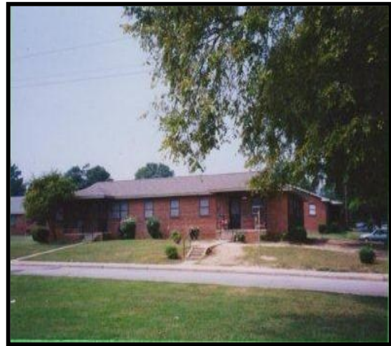
One of the units on the site as it looks today
