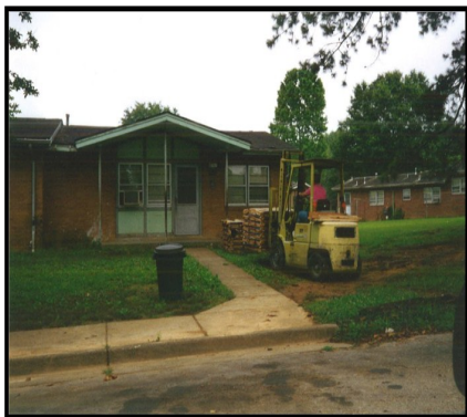
A public housing apartment before undergoing modernization
