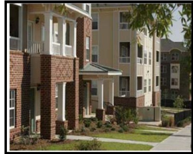
The Ashley CollegeTown mixed-income, mixed-use community was built on the site that once held the Joel C. Harris Homes public housing project.
