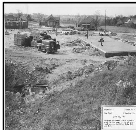
Public housing development under construction in 1962
