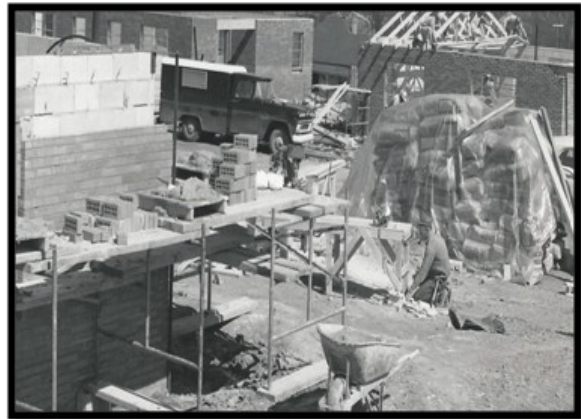
Units on Carver Street under construction, 1963
