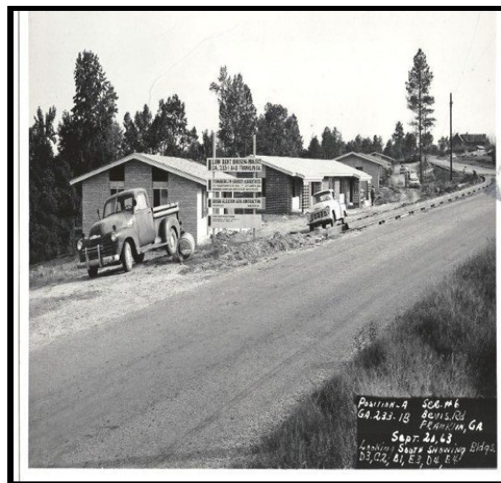
Construction of Robert Canady Homes in 1963
