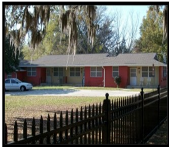
Unit on Gause Street after being renovated
