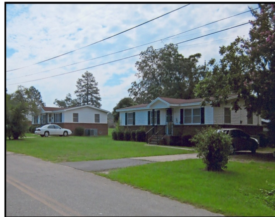
Some of the single family homes owned by the Housing Authority of the City of Ashburn
