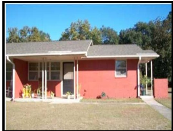
Olive Street property after renovations
