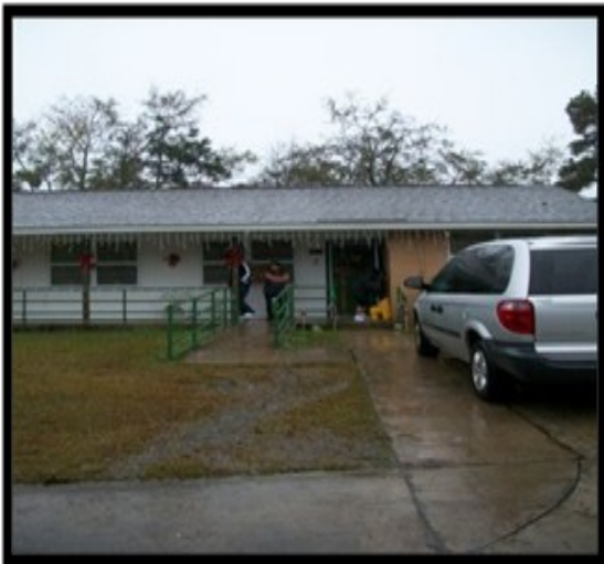
Unit on Gause Street before being renovated
