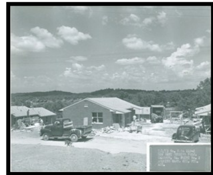
Wylie McDaniel Homes under construction
