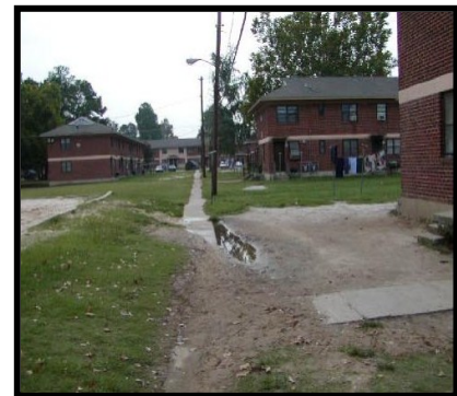
Pictures of George Foster Peabody Apartments before all 510 units were demolished
