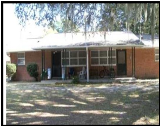
Olive Street property before being renovated
