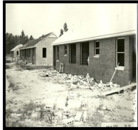
Jim Jones Homes under construction in 1953
