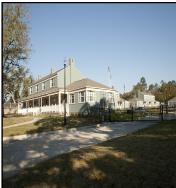
Thronateeska Homes following site improvements in 2011
