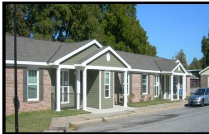
E. J. Knight Homes after major renovations
