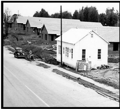
Cannon Homes under construction in 1951
