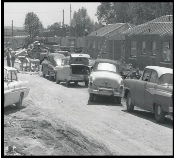
Units on Oak Street under construction in 1963
