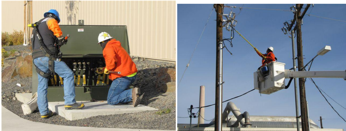
Linemen making repairs to a riser to restore power to 222S/2704S.
