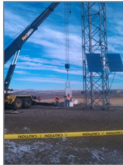
Removal of Equipment from Silo
