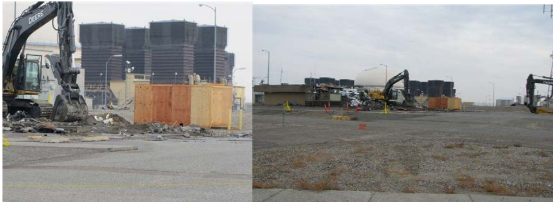
Demolition activities at 4790.
