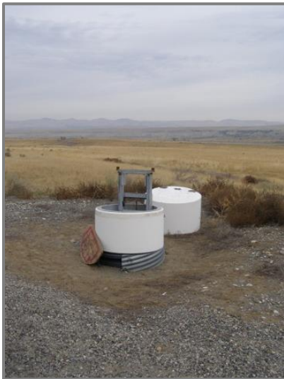
S-8 Siren Silo Pre-Job Appearance
