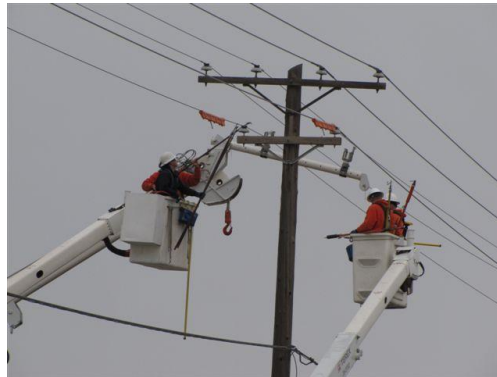
Cross arm replacement.
