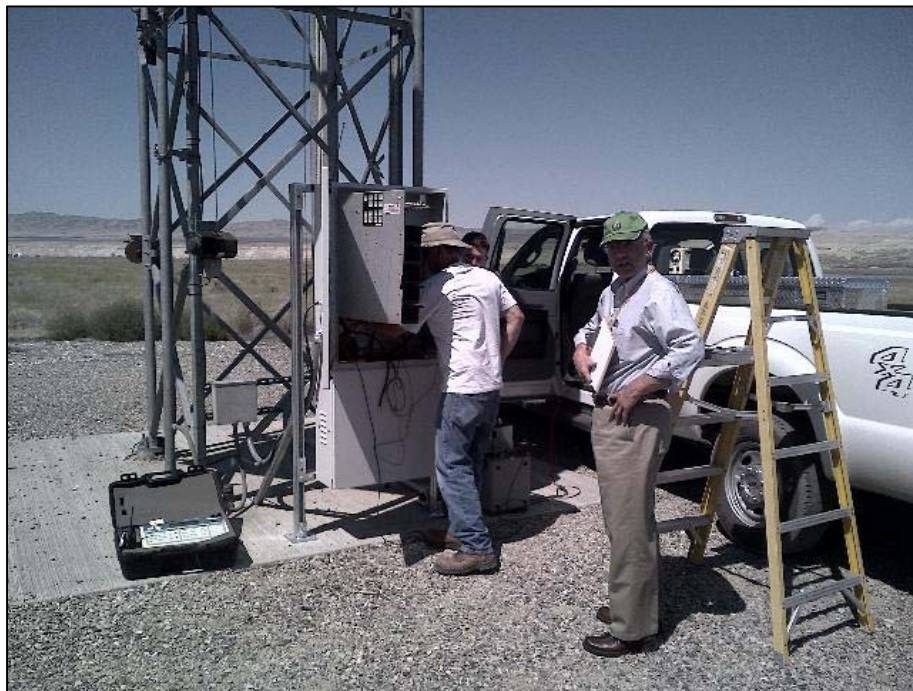
Finalizing the Hanford Site Emergency Alerting System (HSEAS) Siren S8 Work
