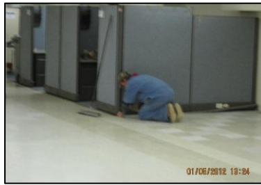
Painters put finishing touches on the vinyl tile flooring installed at MO-287.
