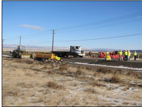
Electrical Utilities Linemen standby to support WCH
