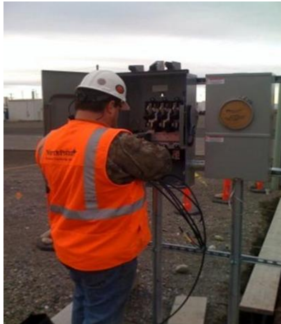
Subcontractor Electrician Working on Meter Rack for 2719WB Digital X-Ray Installation
