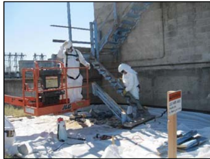
Carpenters begin disassembling the stair case at 182D
