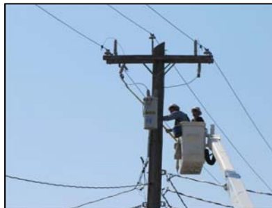
Linemen performing switching evolutions
