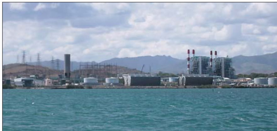
Figure 5.4. Aguirre Power Plant adjacent to Jobos Bay. Photo: NOAA CCMA.
