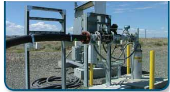
Perched Water Extraction Pilot Test at B Complex
