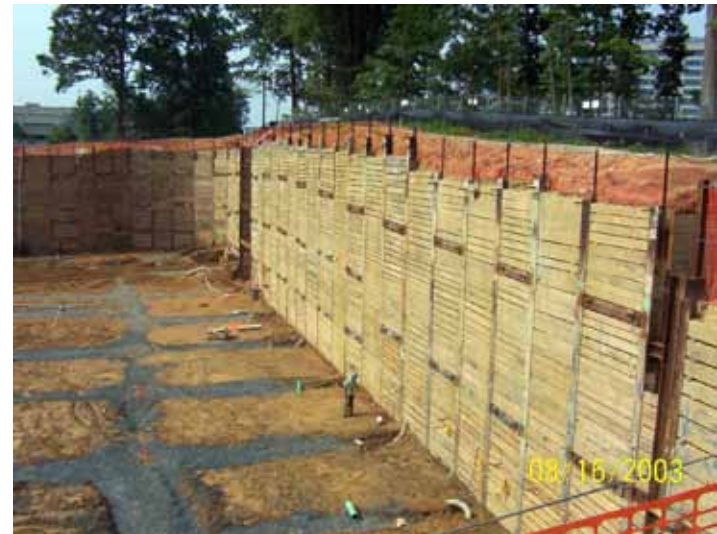
Superior Foundation, Inc.
