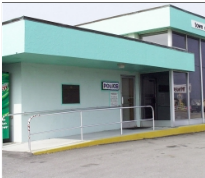
A town chose to alter its police station rather than move its programs and services to another accessible location.
