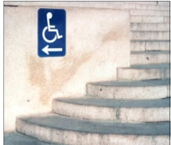
Sign at an inaccessible entrance provides directions to the nearest accessible entrance.
