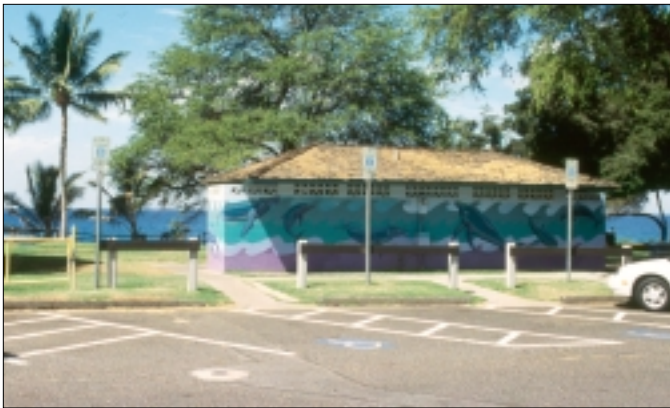
Physical modifications to provide program accessibility included parking spaces, the public toilet facility and an accessible route to the ocean overlook.
