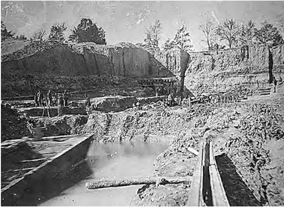
White troops as well as black toiled from August through December 1864 to dig the Dutch Gap Canal, a shortcut for Union shipping to avoid Confederate batteries on the James River.
