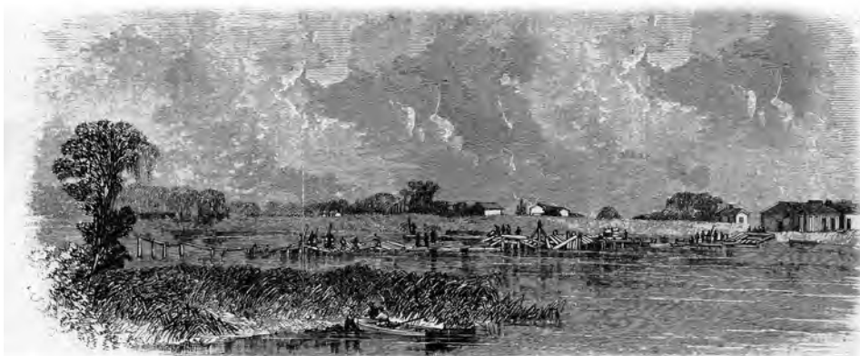
Soldiers from one of the Corps d'Afrique engineer regiments at work along the Bayou Teche in the fall of 1863
