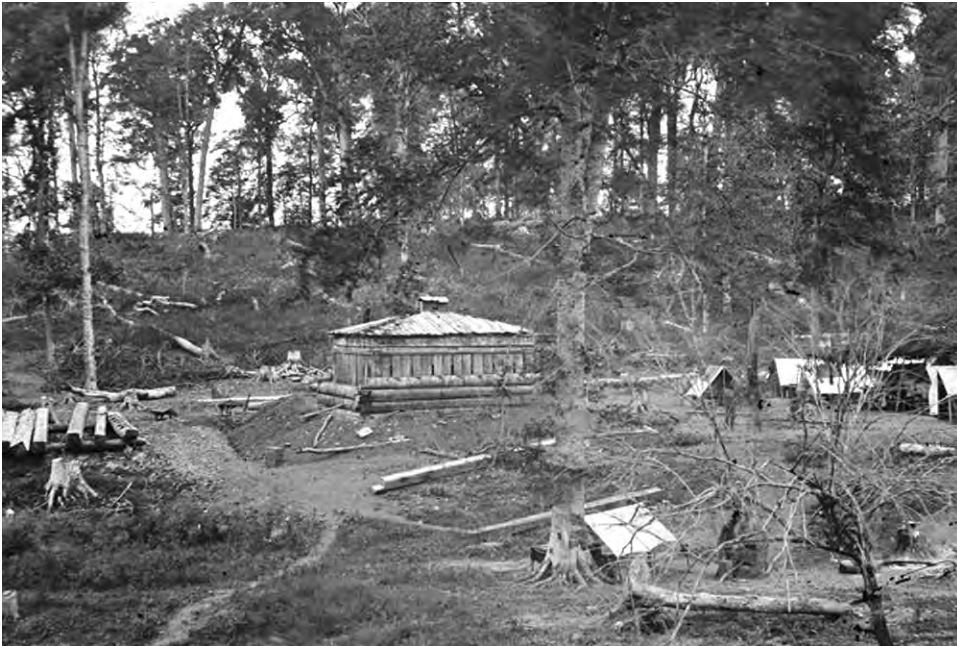
A typical federal blockhouse on the Nashville and Chattanooga Railroad
