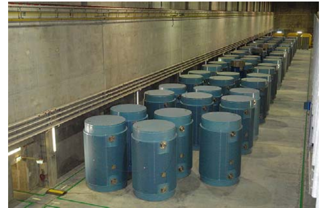
Interim Storage North at Greifswald with CASTOR 440/84 casks containing VVER fuel (photo: EWN)
