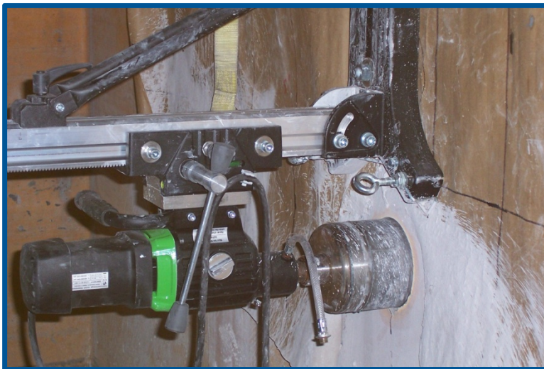
Core Drilling Rig
