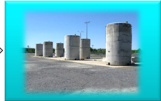
Dry Storage Facility (on site)
