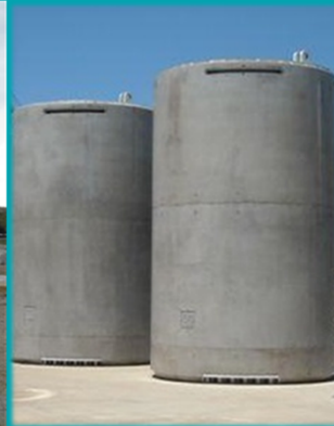
Vertical Concrete Cask At McGuire
