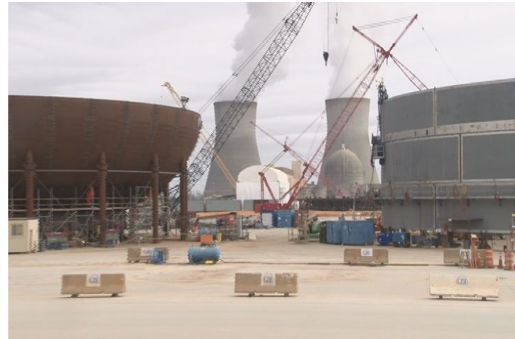
Construction of new nuclear power plant at Vogtle Site
