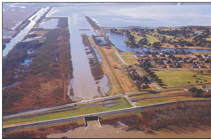
The Caernarvon diversion structure: a potential location of the sediment enrichment demonstration.
