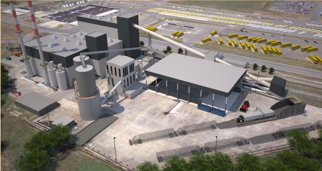
Griffiss Business and Technology Park CHP facility
