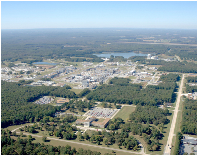
Photo no. D0510264
