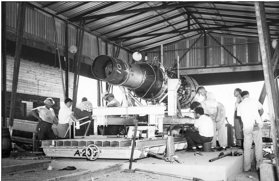
The first jet engine test at AEDC in 1953 required design and construction of a thrust stand for the J47 turbojet engine used in calibrating the T-1 high-altitude test cell. The J47 engine powered the B-47 bomber. (File photo)
