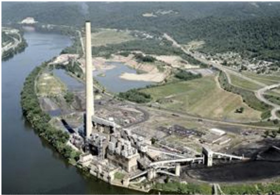
FirstEnergy's R.E. Burger Plant
