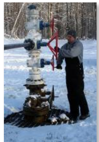
Injection well at Michigan site
