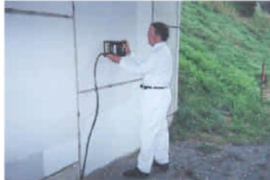
Figure 7. Using GPR to survey a structure
