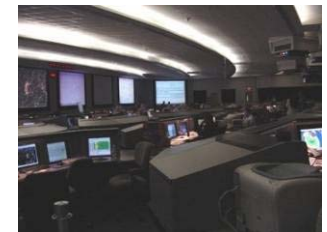
2 Operational Control Centers
